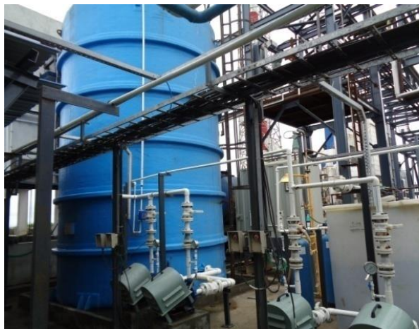
Storage for treated water-STP
