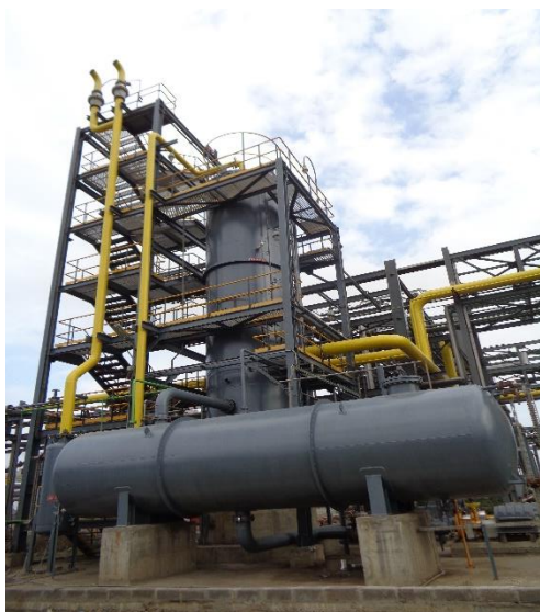
Air pollution control for Boiler
