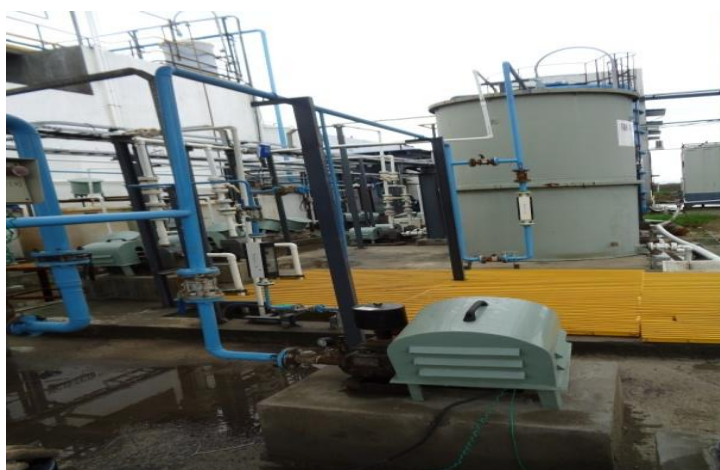
Collection tanks and FAB reactor-STP
