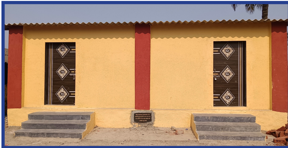
Construction of 2 Classrooms at Zilla Parishad School, at Mazagaon in Patalganga, Maharashtra
