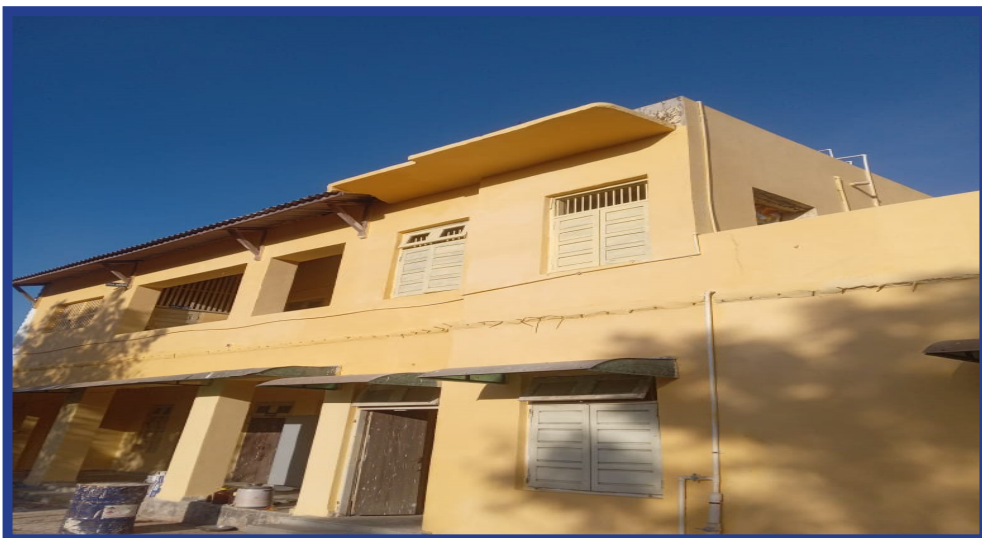
Repairing and painting work done at Boys Hostel at Dahej, Gujarat
